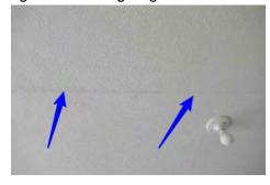
Common concrete cracks in the garage floor.
