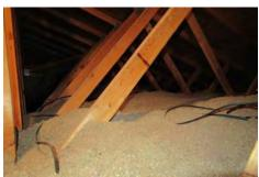
Missing Insulation noticed in the • Hallway attic. Recommend installing insulating in the attic for energy efficiency.
