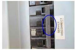
The main electrical panel is missing the safety tag. This takes away the responsibility if anything goes wrong with the meter or incoming electrical lines. Recommend contacting the power company to inspect and install a safety tag.
