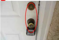
Safety Issue: There is Double Lock Hardware installed on the • Front exterior door. This is a safety concern to be able to exit the home in a timely manner. Recommend replacing double key lock with single key lock for safety.
