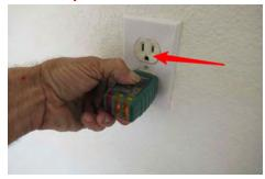
Safety Issue: The • Rear Exterior GFCI outlet Did Not Trip when tested. GFCI's protect against shock or possible serious bodily injury. Recommend replacing the GFCI by a licensed electrician for safety.
