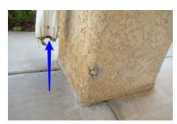
The exhaust vent pipe is starting to Rust. Recommend replacing the vent pipe.
