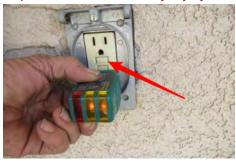
Safety Issue: Broken/Missing Weatherproof Cover on the • Rear exterior outlet(s). This could allow water intrusion and could cause shock or possible serious bodily injury. Recommend installing weatherproof cover(s) for safety.
