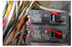
Safety Issue: The • 50 AMP GFCI/ARC Fault Circuit Breaker inside the • Main electrical panel(s) Did Not Trip when tested. This limits the safety protection. Recommend replacing the circuit breaker by a licensed electrician for safety.
