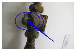
Safety Issue: There Is No Cap on the natural gas line • Behind The Kitchen Stove. The natural gas could get turned on accidentally and this will put natural gas into the livable space. If the natural gas is not being used, recommend installing cap on the natural gas line by a licensed plumber for safety.
