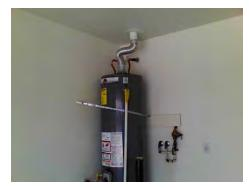
No Expansion Tank was noticed for the house piping. This is a plumbing requirement. Recommend installing an expansion tank.
