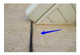
Stucco Damage/Holes were noticed on the • Front
