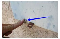
Safety Issue: There is an Open Hole inside the • Main electrical panel(s). If a fire starts inside the electrical panel, the hole(s) could allow the fire to escape through the hole(s) and cause structural damage. Recommend the hole(s) be covered by a licensed electrician for safety.
